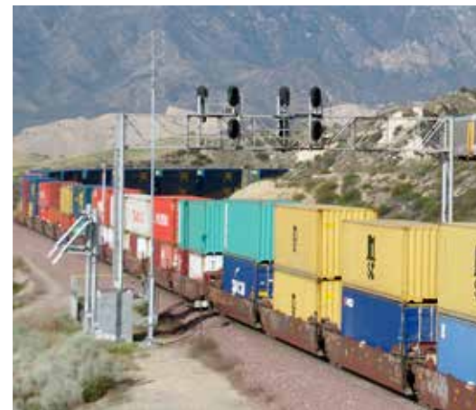
A positive train control radio tower stands next to a signal bridge on the BNSF main line at Cajon Pass. Carl Massart
